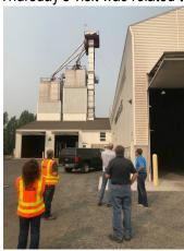
As fertilizer products are transported up the leg, mixed, weighted and dumped into a waiting truck at the Wilbur Ellis facility, observations are made of any fugitive dust. Glen Johnson, Branch Manager in the blue shirt.
